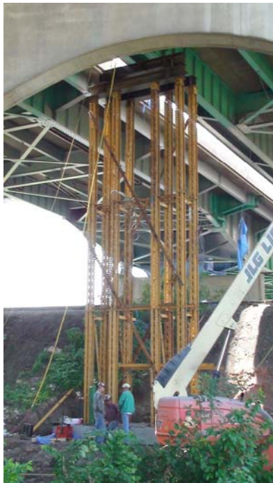
These photographs show the falsework in place under the bridge, the steel beams under the bridge girder and one of the concrete footings.
